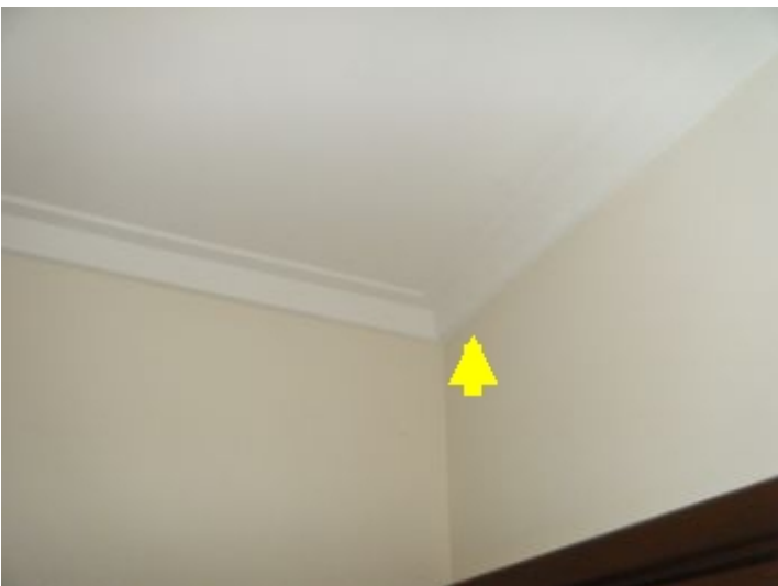
Cornice cracking
